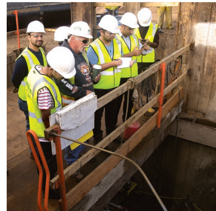
Observing tunnel boring at pump station project in Middletown, CT
