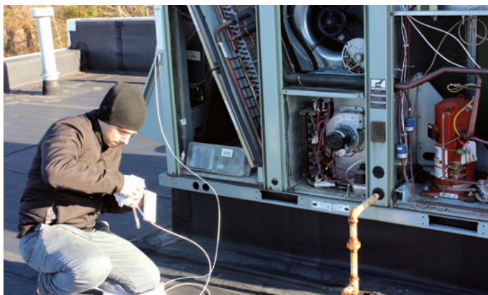
Malak Souissi installing sensors and FDD on rooftop AC unit
